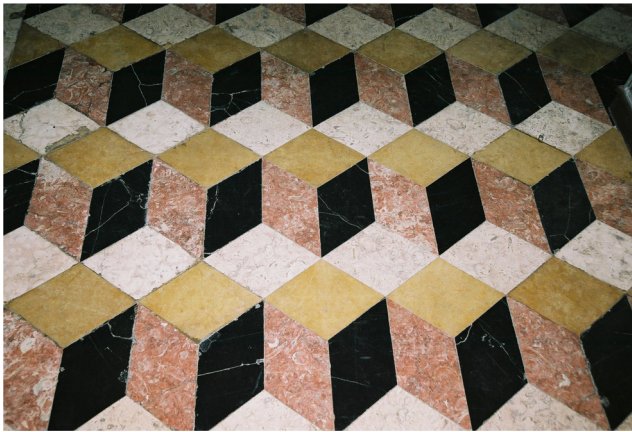
Fig. 15 Pavement of Sacristy, N.S. Carmo Church
