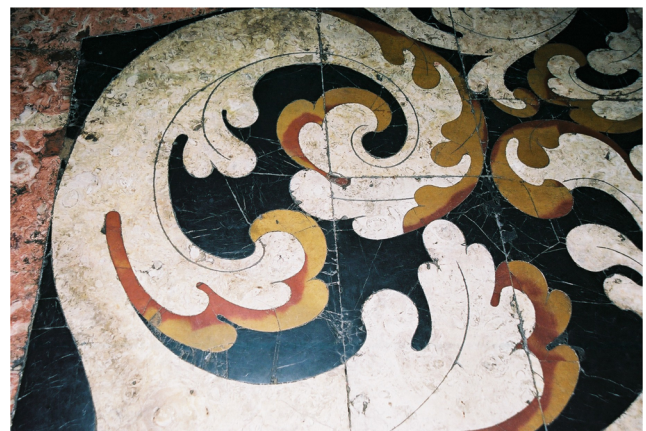
Fig. 18 Lio z inlay at the main altar pavement at São Francisco church in Bahia, Brazil
