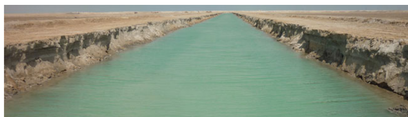
Fig. 6 Newly excavated fish-farm channel in the upper intertidal zone. Such channels prevent the flow of subsurface brines in the sabkha system. The width of the channel is 40 m with banks that are 2.5 m high, water depth varies due to localised slumping but rarely exceeds 1 m
