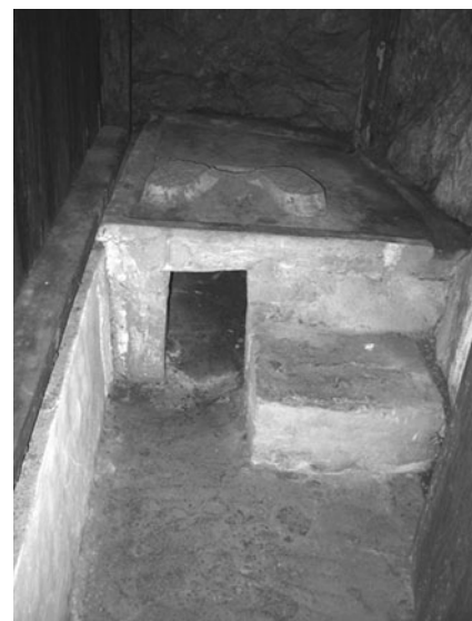
Fig. 7 Asian-style toilets installed in caves at Viengxai suggest the disposal of human faeces directly into cave environments
