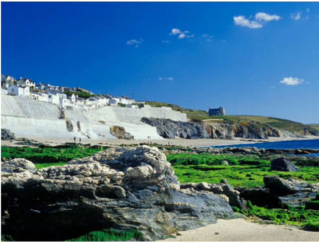
Fig. 5 Concrete sea wall, Porthleven, Cornwall, England. Increased demands for similar coastal protection schemes, constructed in response to coastal erosion, will result in further losses of cliff exposures. Photograph: Mick Murphy/Natural England
