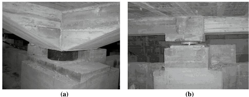
Fig. 5 Bearings mounted in Solarino base isolation system: a HDRB, b LFSB
