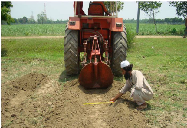
Fig. 7 Paired row trencher during operation
