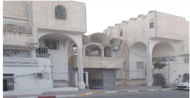
Fig. 6 Second case study external view
