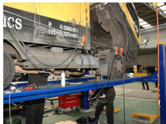
Figure 3. Diesel to LPG engine conversion work.
