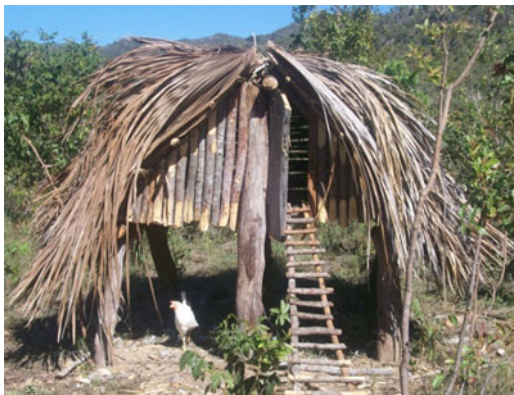
Fig. 6. Roof of a chicken house made with buriti leaves. Engenho II, Cavalcante-GO.
