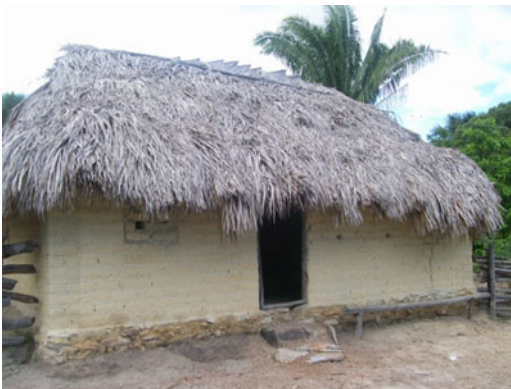
Fig. 1. Kalunga home built with adobe walls using buriti and indaiá leaves for roofing. Engenho II community, Cavalcante-GO.
