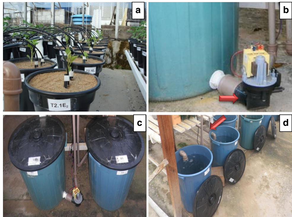
Fig. 3 Irrigation details in the three-phase hydroponic system: lateral pipings with microtubes (a), connection from reservoir to the pump (b), output for irrigation (c), and return system of nutrient solution (d)
