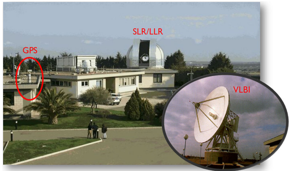
Fig. 1 The fundamental geodetic station “G. Colombo” at Matera, Italy. The three main space geodetic observing techniques are highlighted by labels next to their respective sensors
