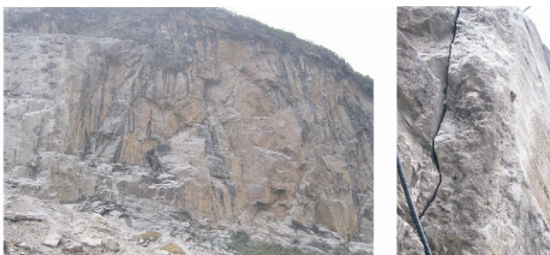
(a) Overall aspect (b) Local crack
