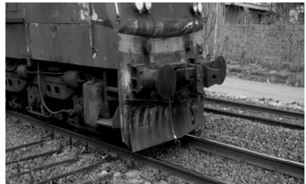
(a) Track with concrete sleepers
