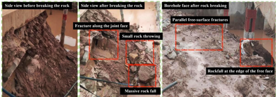
Fig. 15. On-Site Rock Breaking Pictures
