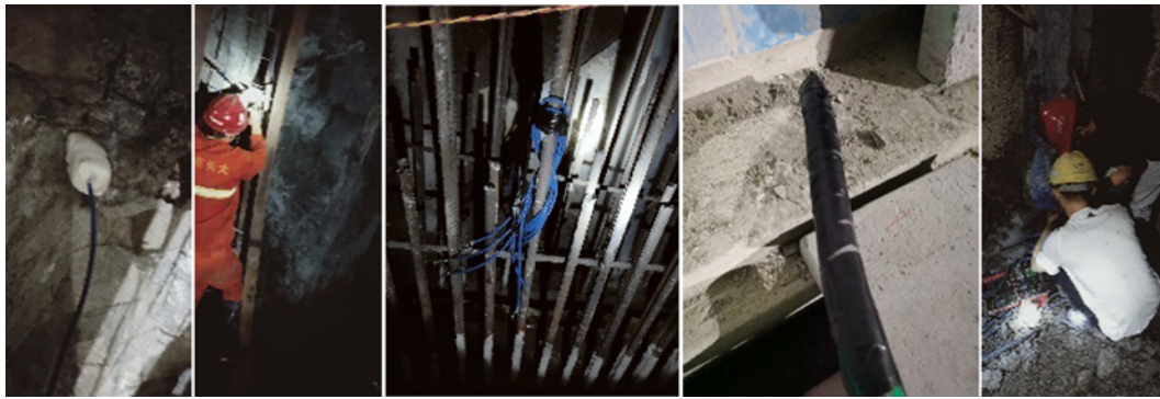
Fig. 9. Embedding and Measurement of the Seepage Pressure
