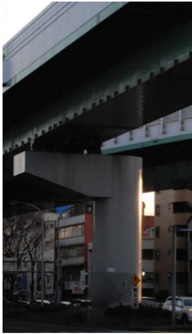
Fig. 1. Eccentrically Loaded Steel Bridge Pier (the inverted L-shaped bridge pier)
