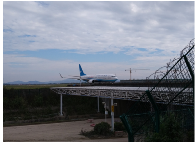
Fig. 4. Taxiway Bridge V
