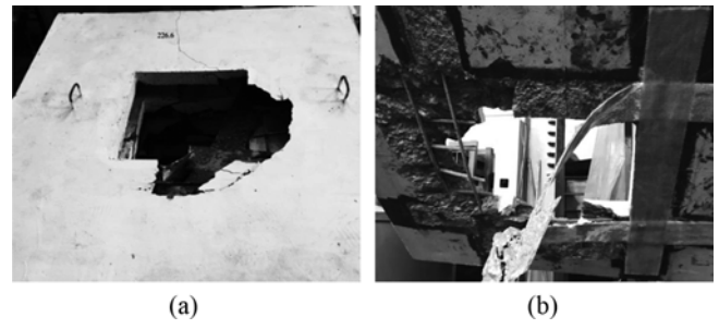
Fig. 12. The Failure Mode and Cracking Pattern for Slab SOGM2: (a) Compression Side, (b) Tension Side
