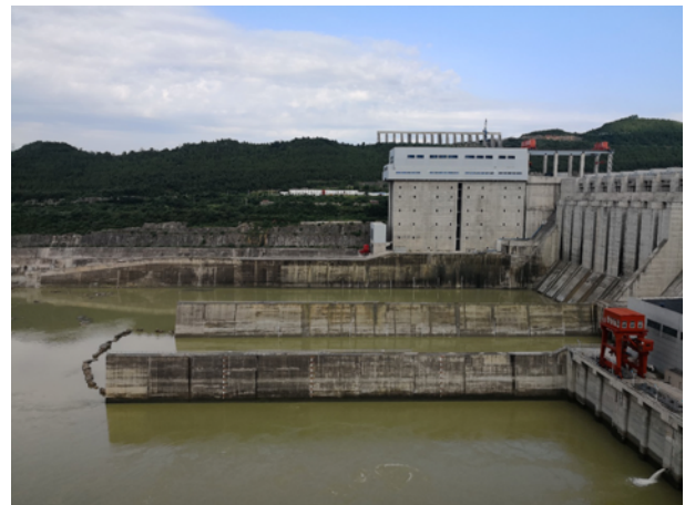
Fig. 1. A Hydropower Station
