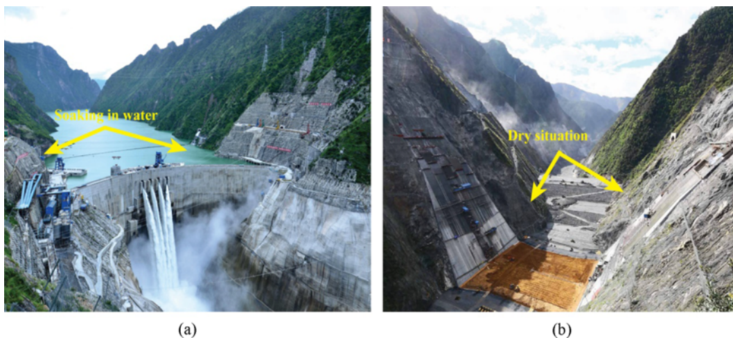
Fig. 1. Rock Mass in Dry and Saturated Condition: (a) Example of Jinping Hydropower Station in Sichuan, China, (b) Example of Lianghekou Hydropower Station in Sichuan, China
