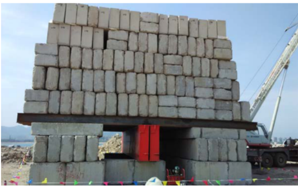
Fig. 5. Concrete Blocks and Reaction System of Static Load Test
