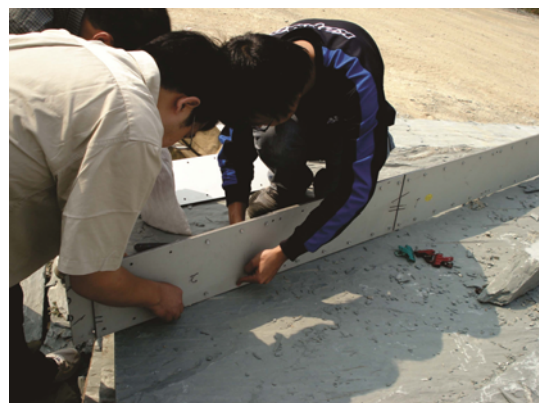
Fig. 2. Installation of the Fixed Boards for Measuring Field-scale Roughness Profiles
