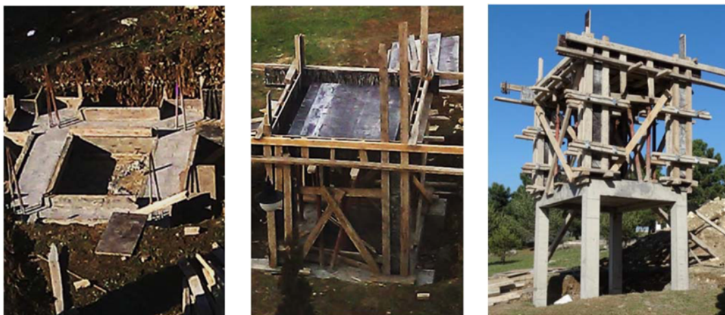
Fig. 1. Construction Phases of RC Field Test Structure
