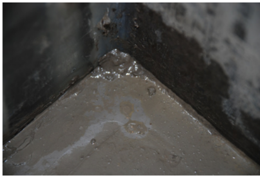
Fig. 3. Sand Piping at the Corner
