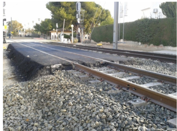
Fig. 1. Detail of the 20 m Stretch of Asphalt Slab Track Inserted between the Previously Existing Concrete Slab Track and Ballasted Track
