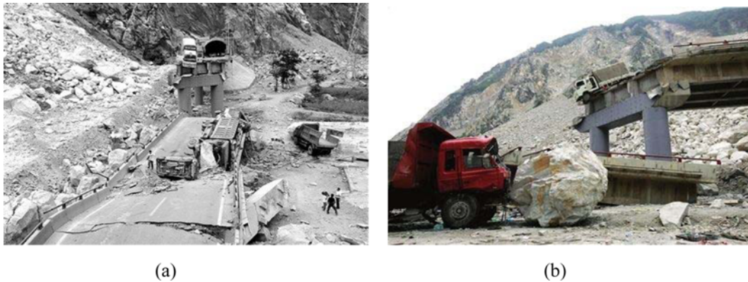
Fig. 1. A rockfall Disaster Occurred in Yingwen Road of China: (a) The Damaged Bridge, (b) The Falling Rock
