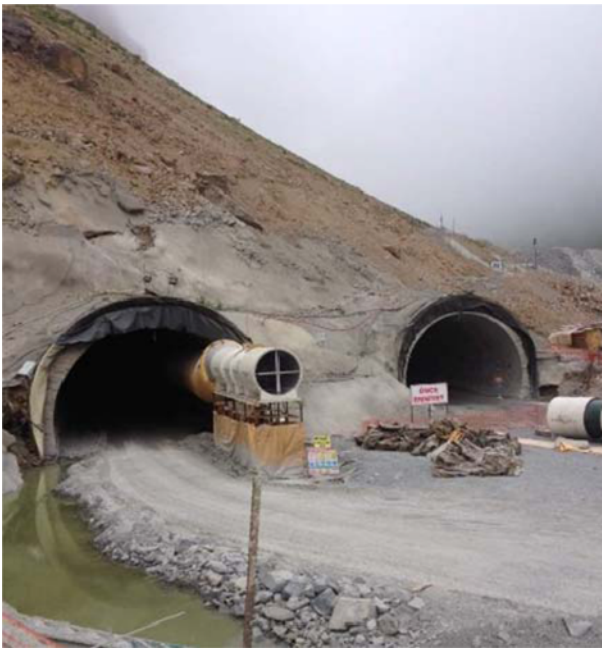
Fig. 1. General View of the OMT Portal
