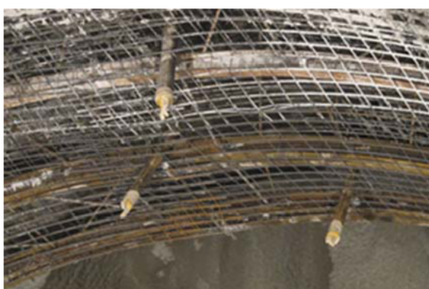
Fig. 8. Support Installation in the OMT
