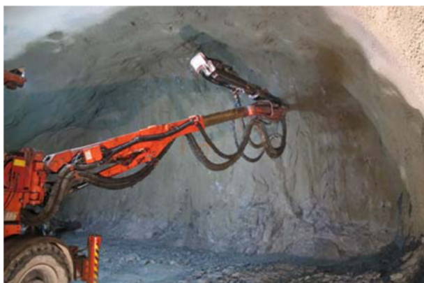
Fig. 7. Wheel-mounted Drilling Rig
