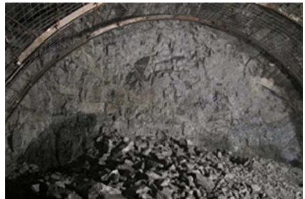
Fig. 6. The Placement of the Steel Wire After the Excavation Process
