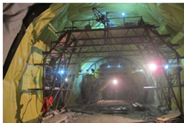
Fig. 9. Waterproofing Installation at OMT
