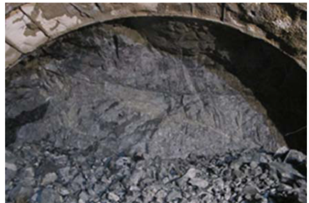
Fig. 5. Prepared Site for Tunnel Excavation
