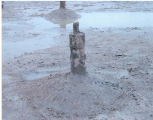
Fig. 3. Micropile after Installation
