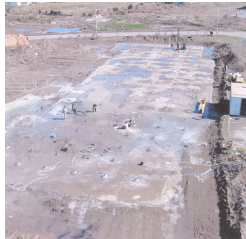
Fig. 5. Plan of Micropile Installation (KHANEH DARYA Complex)
