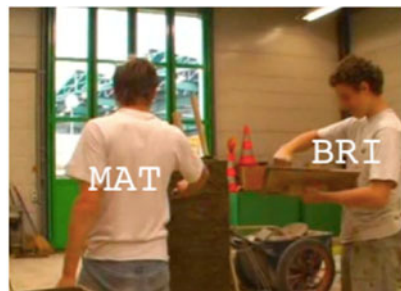
#2: MAT approaches the wall and shows BRI how to throw cement
