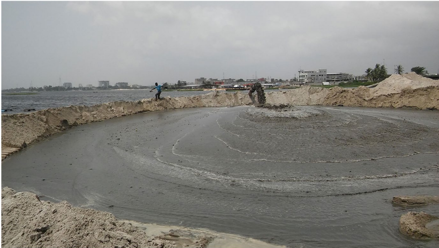
Figure 5 Land reclamation at Soweto Remblais with water and sand pumped by digger boats. Source: author
