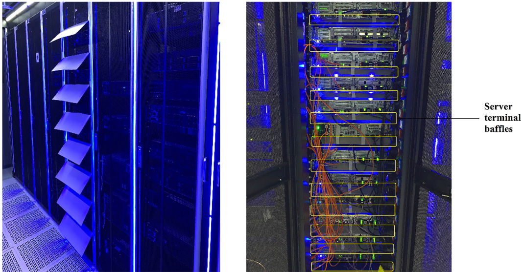
Fig. 7 Installation of rack baffles (left) and server terminal baffles (right)
