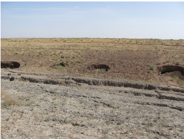
Figure 8. The collapsing sinkholes in downstream of dyke D situated along the border of subsidence band.
