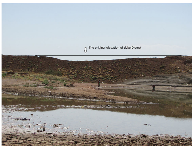
Figure 6. The extra settlement of dyke D crest (view from basin toward the dam).
