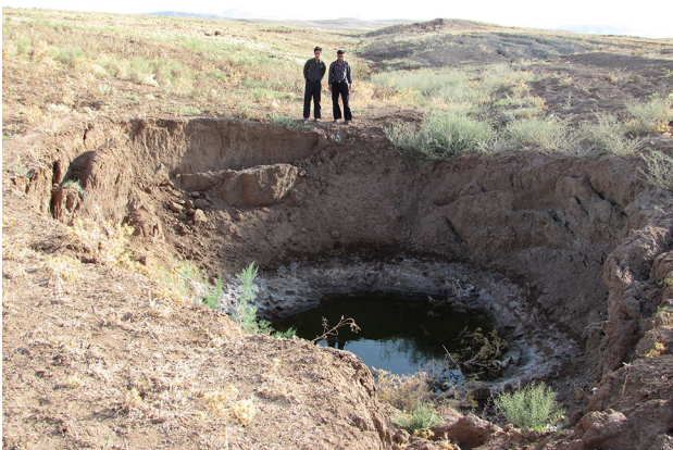
Figure 9. The opening of largest collapsed sinkholes in downstream of dyke D.
