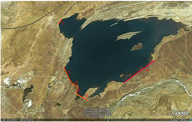
Figure 2. The plan view of Arbatan reservoir in full condition and circumference dykes.
