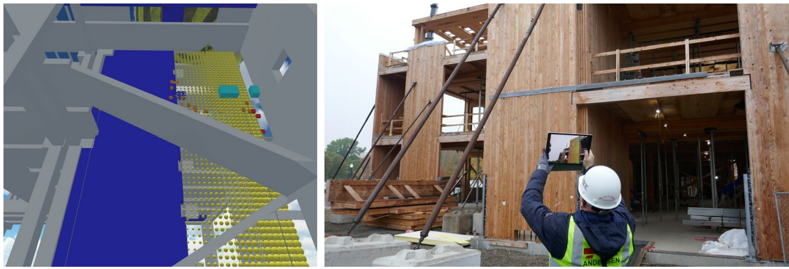
Fig. 5 Example of representing data with a particle system in both the virtual reality (a) and augmented reality setups (b). The size of the particles is proportional to the moisture content of the CLT panel
