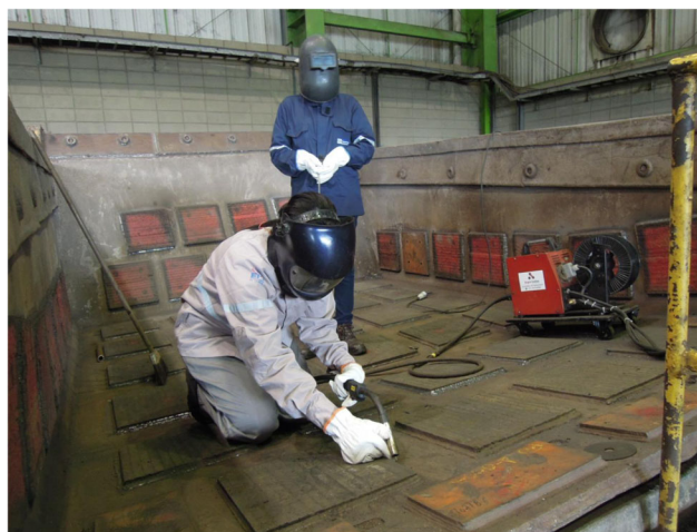
Fig. 2 Mock-up showing the relative positions of the welder and the sample taker who operates the bellows pump. The plastic tube connects the bellows pump to the sample tube. The geometry provides flexibility to the welder for rapid movement to avoid unexpected safety risks such as spatter of molten metal
