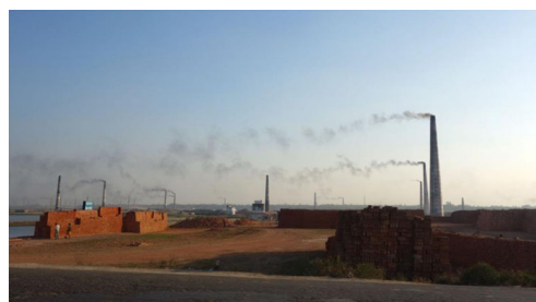
Fig. 2 Cluster of fixed chimney brick kilns in operation in the Greater Dhaka region (photographed by Dr. Khaliquzzaman)
