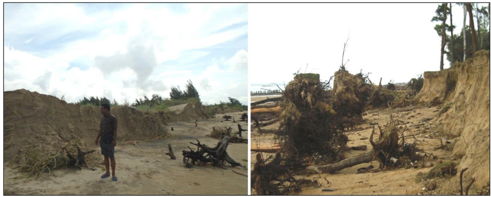
Plate 4 Increased rate of beach cliffing and cliff recession along the shoreline of Jaldha mouth and Sankarpur due to the pressure of high tidal prisms
