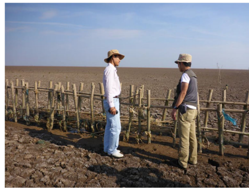
Fig. 2 Low-cost bamboo breakwaters, which have lost most of inner-grass fences. Photo taken at Soc Trang province in the Mekong Delta, March 2014
