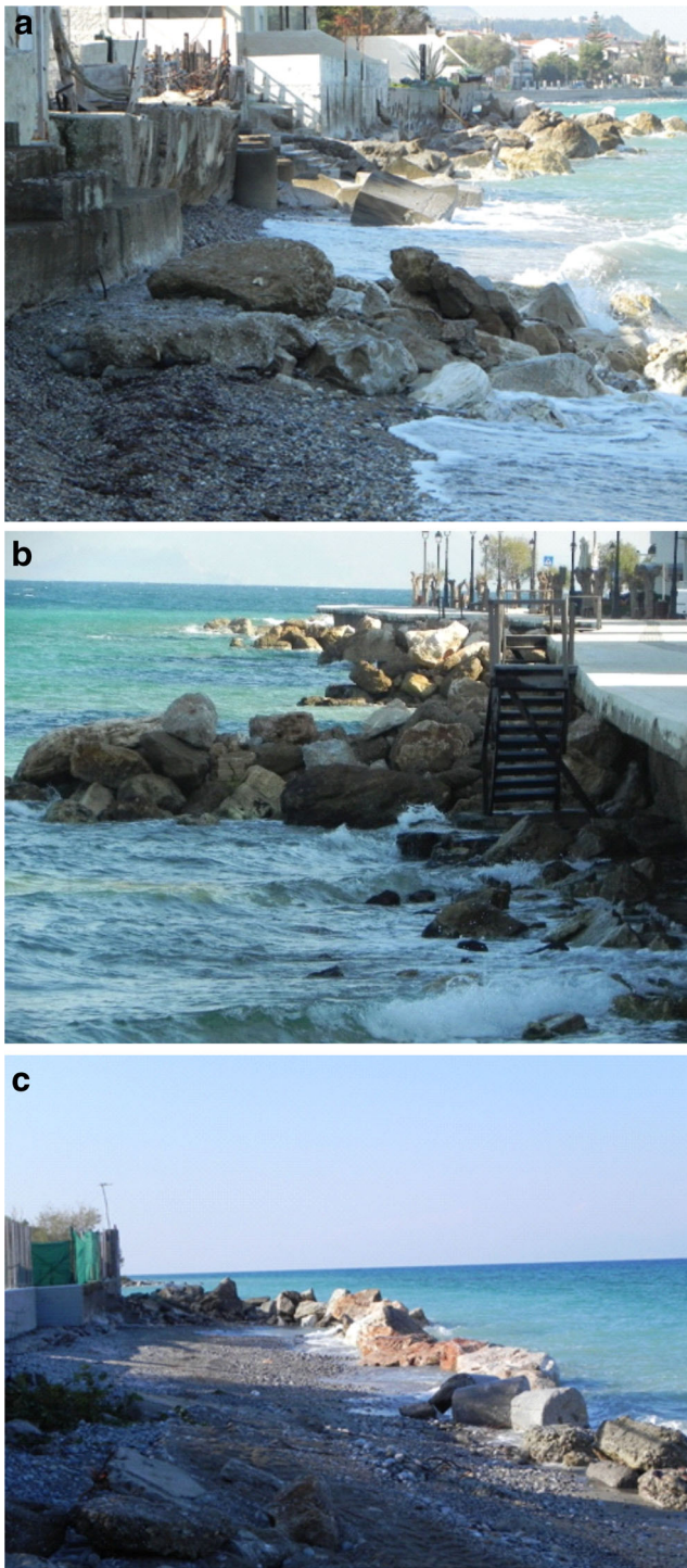
Fig. 5 a Break water piers using natural boulders across the waterfront of Sykea village do seem to have reduced the retrogradation phenomenon but an average of 20 m of coastal zone has been lost in a 72-year period. b Several measures and constructions along the Xilokastro waterfront have slowed down the coastal erosion that reached the rate of 0.66 m/year for the study time period. c The highest rates of retrogradation were calculated along the Kamari beachfront where serious damages are expected the next few years, as no serious measures have been taken for the coastal conservation. See Fig. 1 for the locations of the photographs
