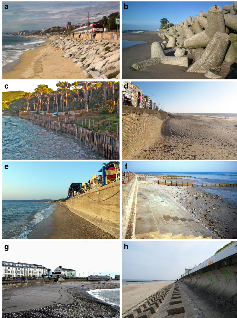
Fig. 4 Structures adherent to the coast. a Revetment (El Masnou, Spain); b Rip-rap in tetrapods (Poland); c Wooden seawall (Punta Ala, Italy); d Masonry seawall (Koksijde Bad, Belgium); e Linear concrete seawall, Glifoneri, Kasandra Peninsula, Greece); f Stepped seawall (Channel coast, UK); g Seawalls with tarmacadam pavement (Porthcawl, UK); h Concrete concave seawall with lower rough surface (Poland)
