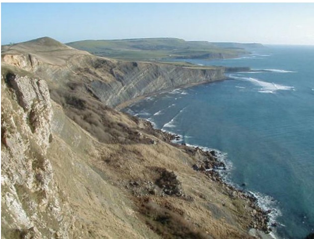
Fig. 3 Purbeck coast (Source: Author 30th December 2001) Vertical limestone cliffs with incipient toppling in left foreground. Middle slope partially exposed Kimmeridgian shales with back-tilted failure block with scrub, maritime grasses and wind-modified woodland. Marine erosion retarded by boulder arcs. Middle ground: vertical cliffs in shales and clays with offshore ledges (part of marine reserve). Kimmeridge Bay beyond has high importance for Kimmeridgian fossils. Public access limited to cliff-top path
