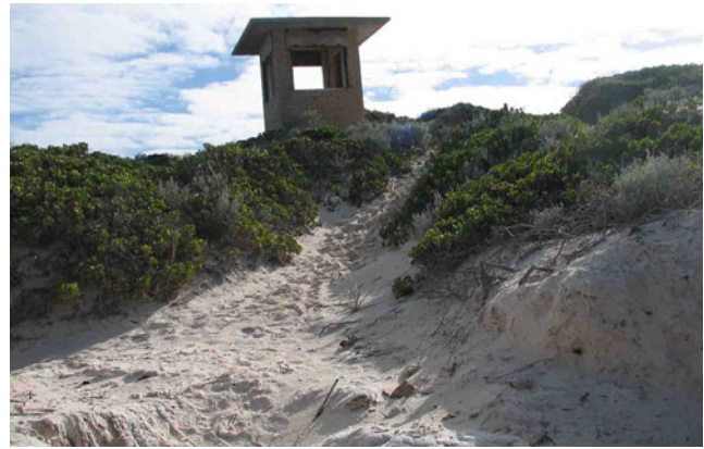
Fig. 8 Devegetated and eroded foredunes from foot traffic on the northern side of the vehicle access at the 'Sentry Post' (see Fig. 1 for location) south of Wedge Island settlement
