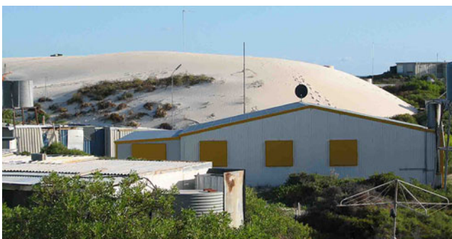
Fig. 4 Foredune blowout at Grey Shack Settlement overwhelming coastal shacks, looking north
