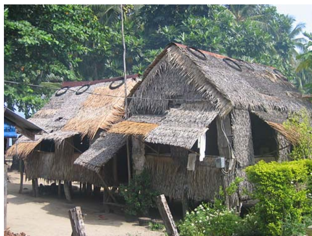
Fig. 3 Traditional house made of bamboo and palm leaves on the island of Divinubo, Borongan, Philippines (photograph by JC Gaillard, August 2006)
