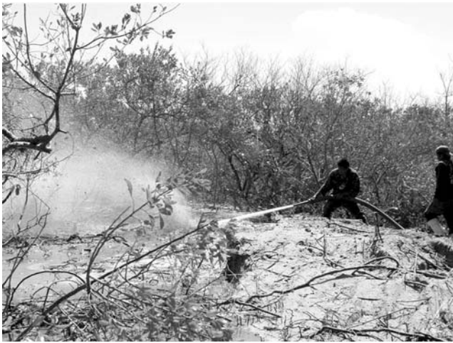
Fig. 2 This photo shows a hydro-leveling crew in action. Water under high pressure is jetted onto the spoil mound and the material is washed into the adjacent wetlands
