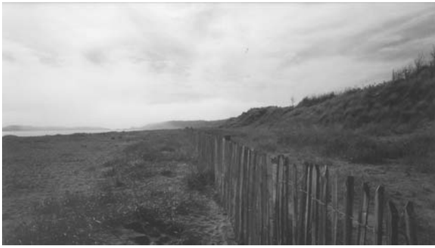
Fig. 11 Frontal dune accretion aided by fencing, Traeth Llanddwyn, Newborough, looking west-northwest (taken in 2000)
