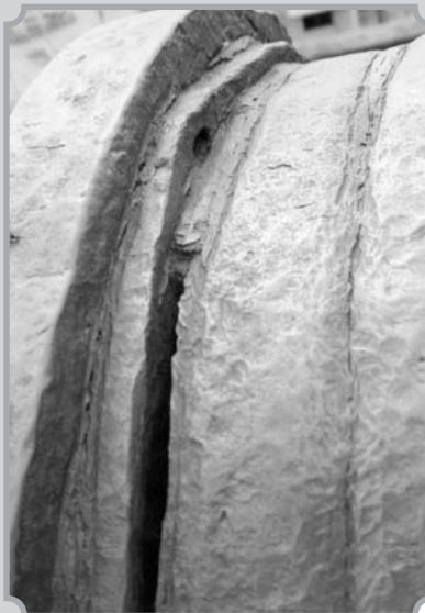
Figure A. A close-up view of one of the forge-welded joint regions on the outer surface showing that a smaller ring has been used to join the gaps between larger rings. The provision of a handling hole on the smaller ring should also be noted.
