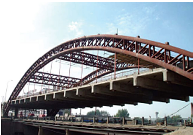
Fig. 7 Xining Beichuan Arch Bridge [71]
