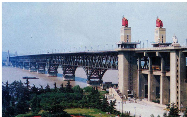
Fig. 6 Figures 1, 2, 3, 4, 5, 6, 7, 8, 9, 10, 11, 12, 13, 14, 15, 16 and 17 A photograph of the NYR steel truss bridge [56]
