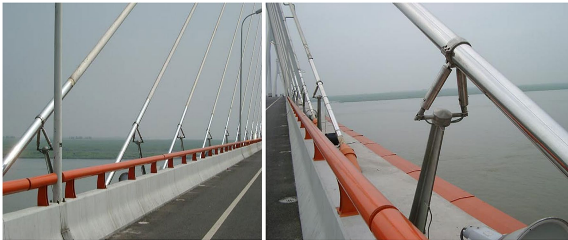
Fig. 14 Semi-active MR dampers installed on the Dongting Lake Bridge
