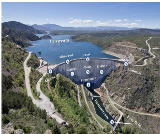
Fig. 10 a A disposition of the installed sensors in a dam. b Flow diagram of DM data analysis
