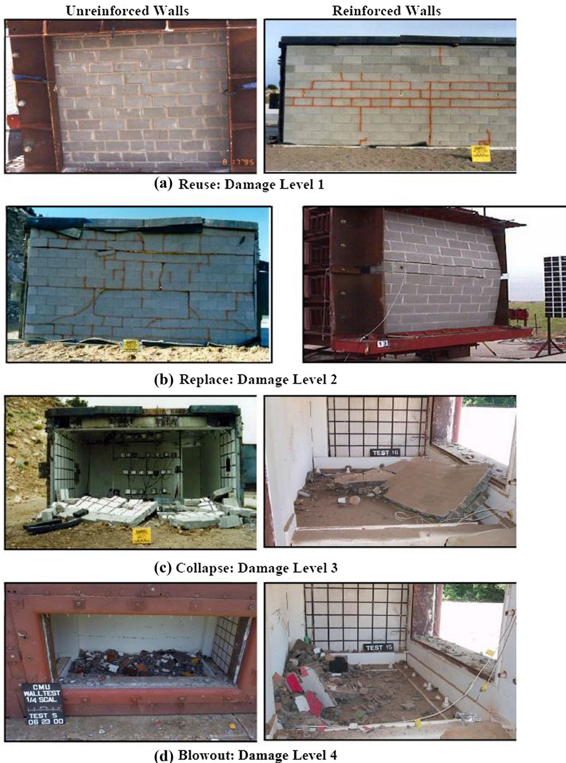
Fig. 40 Wall damage classifications in the Wesevich and Oswald study [152]
