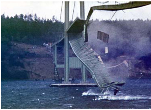
Fig. 1 The collapse of the Tacoma Narrows Bridge on 7 November 1940
